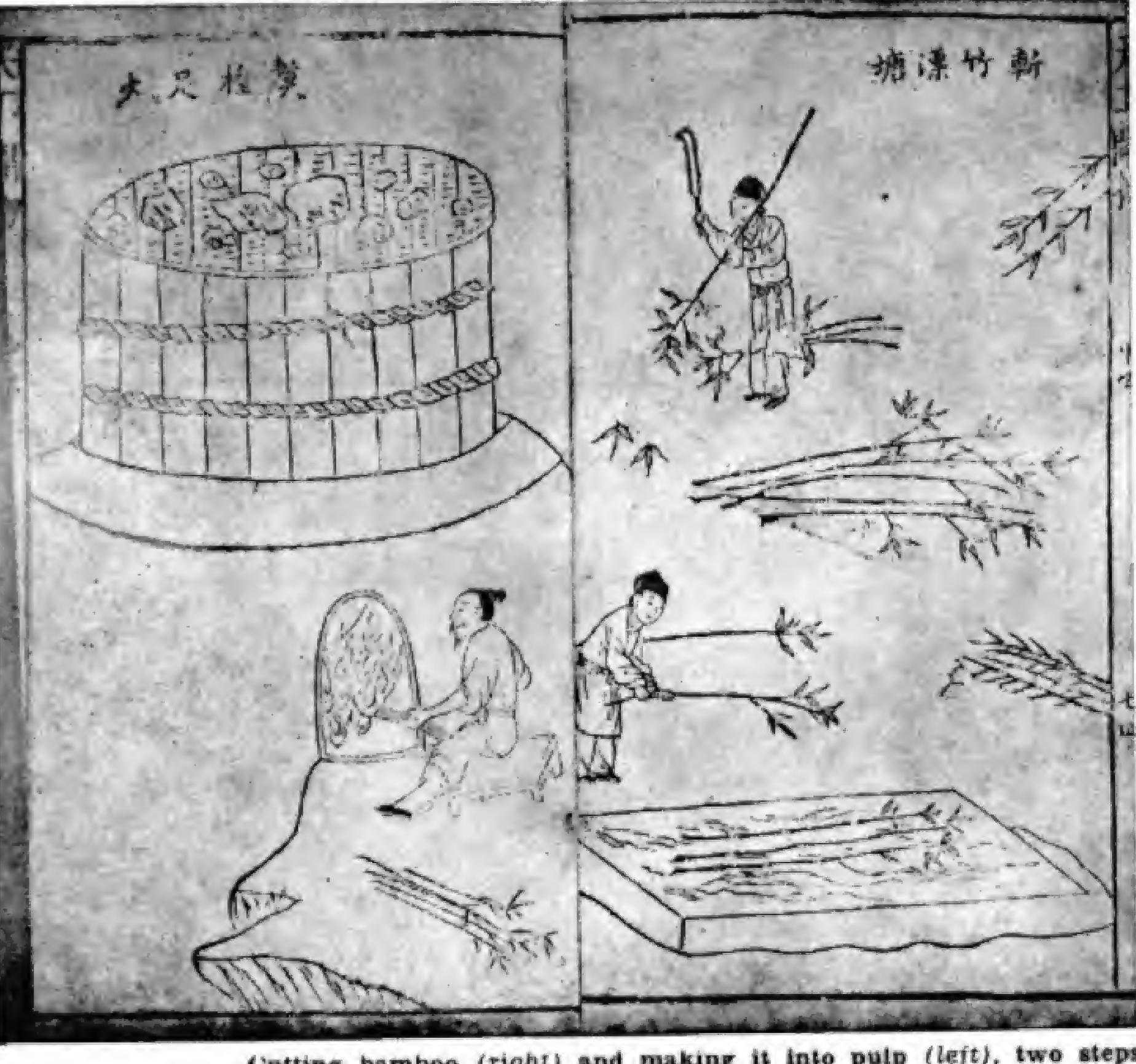
Cutting bamboo (right) and making it into pulp (left), two steps of the handleraft paper-making method as shown in Tien Kung Kai Wu, an early Chinese technological treatise printed in 1637.
